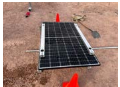
PHOTO 9: IR-30 system after compressive load tests
