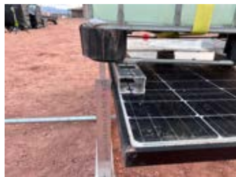
PHOTO 8: Slight deflection noted under load
