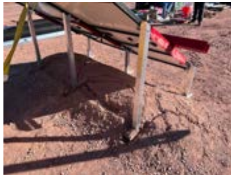
PHOTO 14: Ballast and frame after completion of testing
