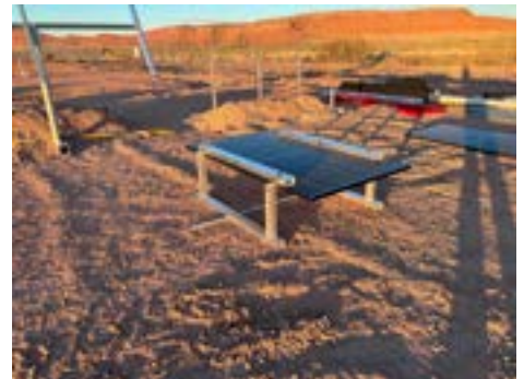
PHOTO 3: IR-30 Solar Racking System setup for test
