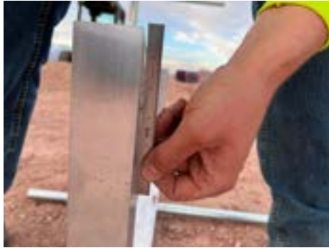
PHOTO 10: Slight deformation after load removed
