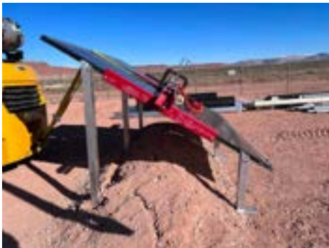
PHOTO 13: Ballast after completion of testing
