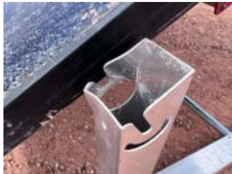
PHOTO 14: Upright mount deformation after testing
