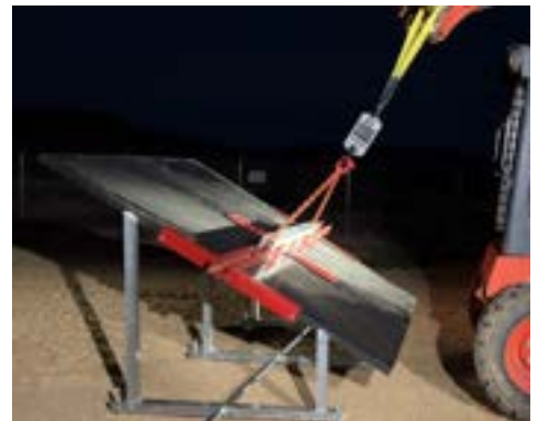
PHOTO 6: Test setup - IR-30 Solar Racking System with AnchorSpikes
