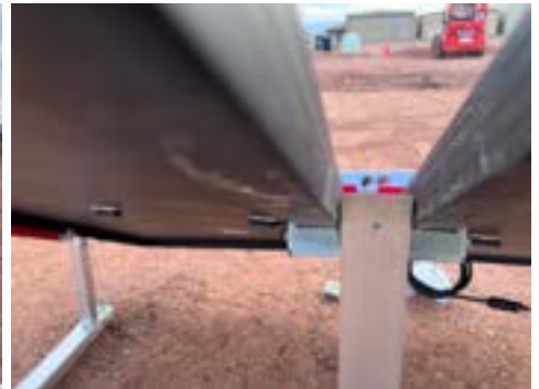
PHOTO 12: Middle brackets after testing
