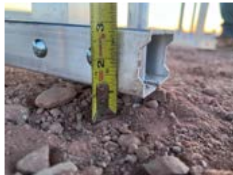
PHOTO 5: Ground to frame measurement example at Spike #3
