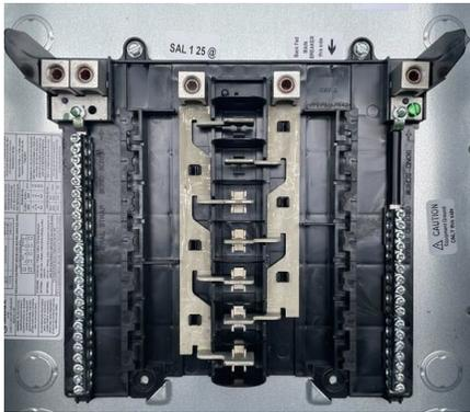
**Figure B - Typical Main-Lug-Only Electrical Panel Busing**
