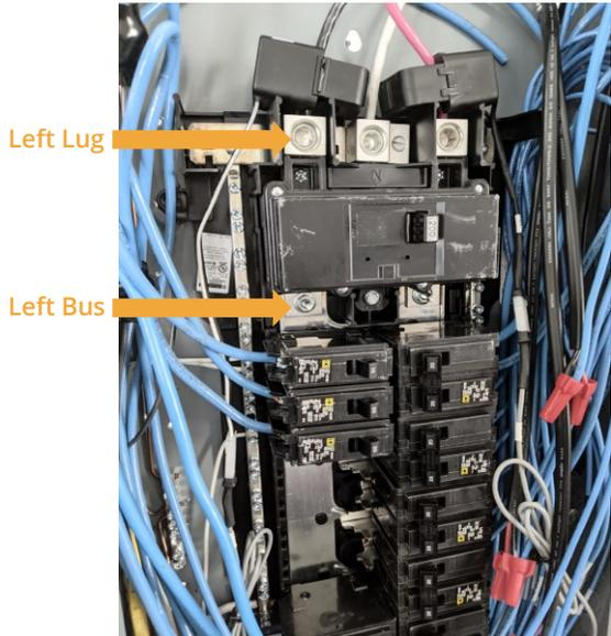
Figure C – Typical Main Breaker Electrical Panel
